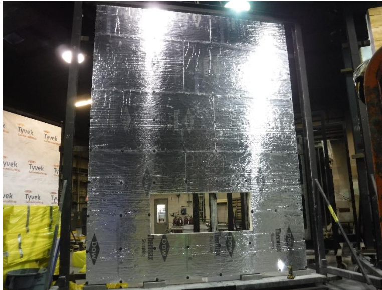
Photo No. 3 DuPont™ Thermax™ Installed
