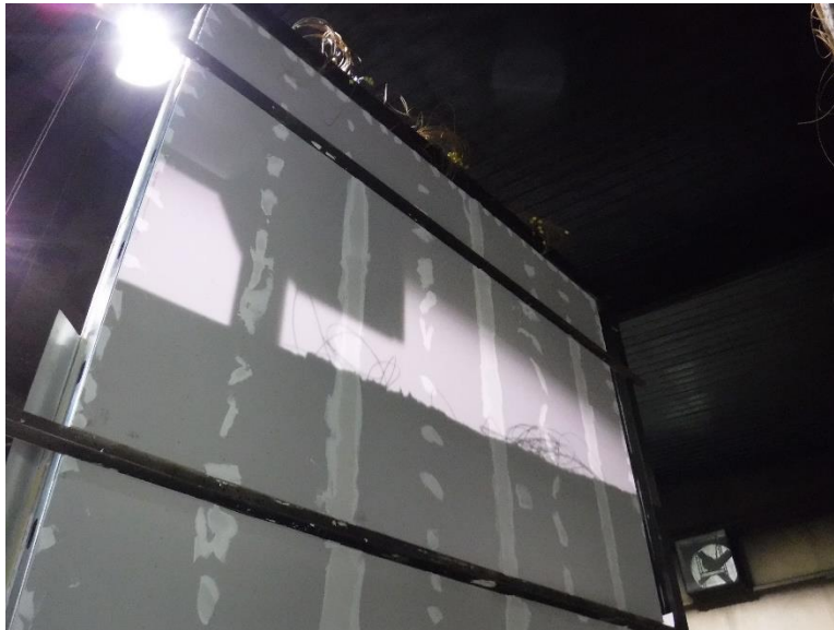
Photo No. 8 Second Story Interior Gypsum (Pre-test)
