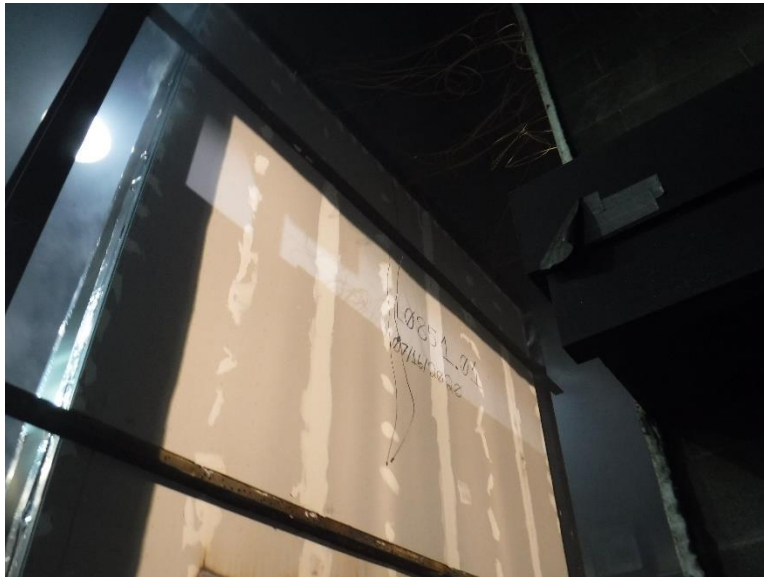
Photo No. 16 Second Story Interior Gypsum (Post-test)
