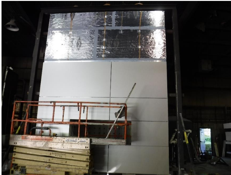
Photo No. 6 Panel Installation
