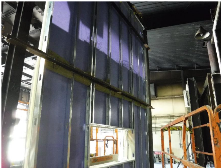
Photo No. 2 Exterior Sheathing and Siding Completed
