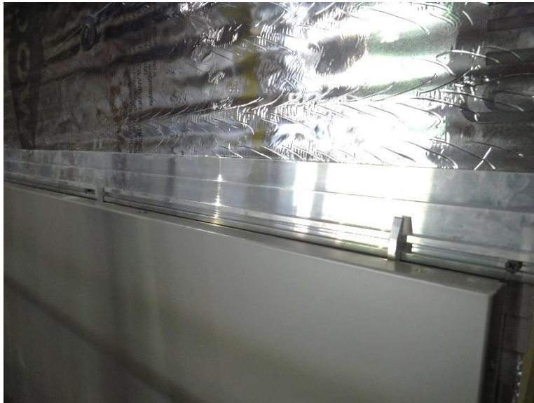
Photo No. 4 Typical Panel Attachment to Aluminum Extrusions
