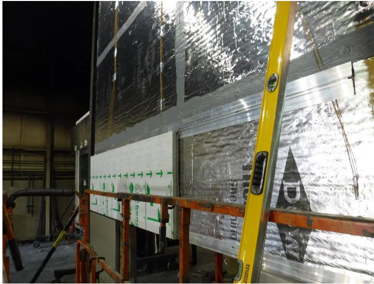
Photo No. 5 Panel Installation Above the Window Opening
