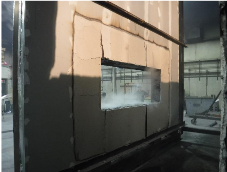
Photo No. 15 First Story Interior Gypsum (Post-test)
